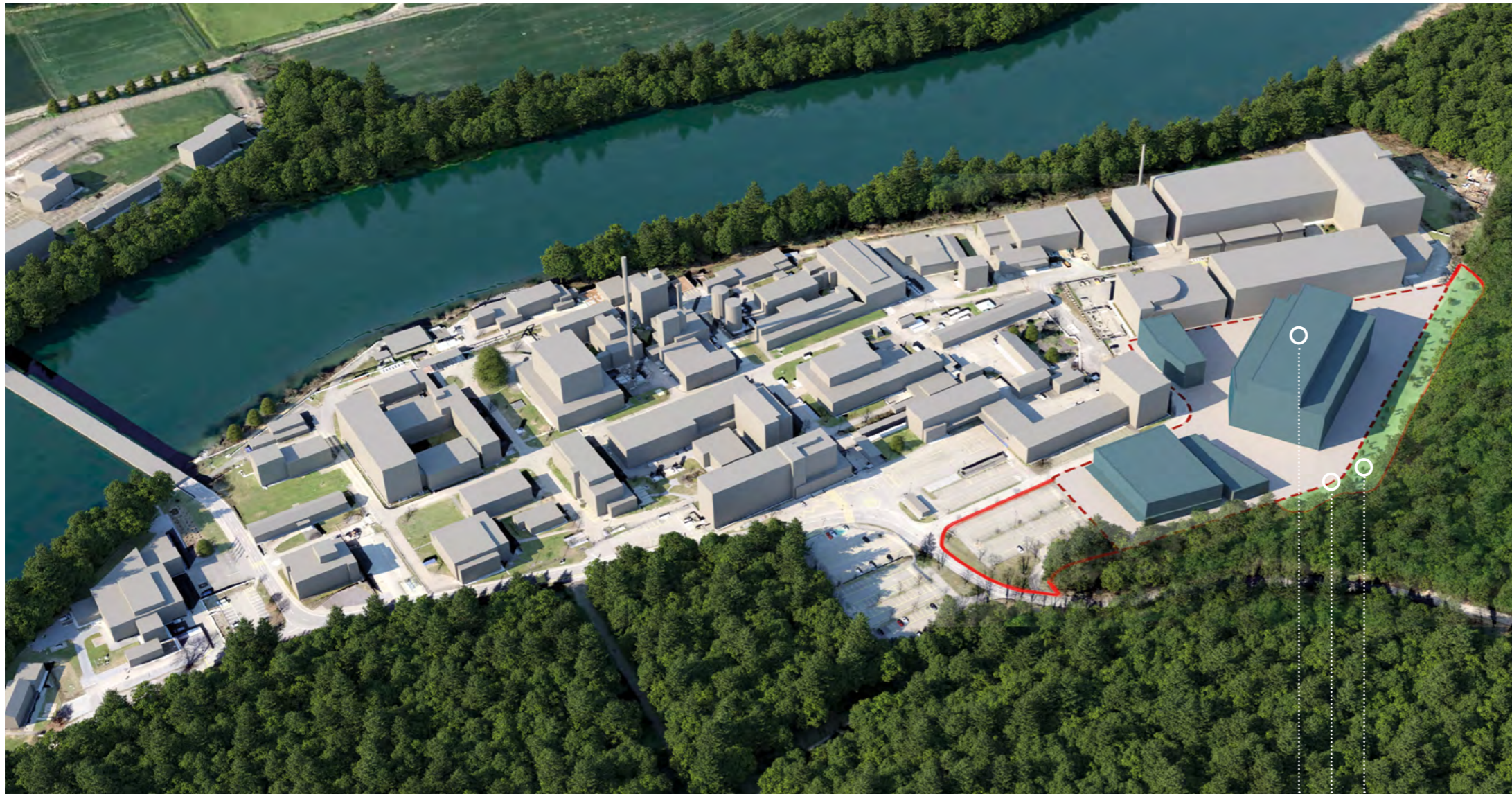
The encapsulation plant for spent fuel assemblies will be constructed at the site of the Zvilag interim storage facility.
